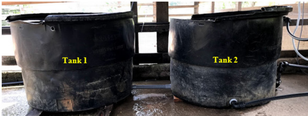
Figure 2. A two-tanks system was applied to ensure a continuous supply of water
